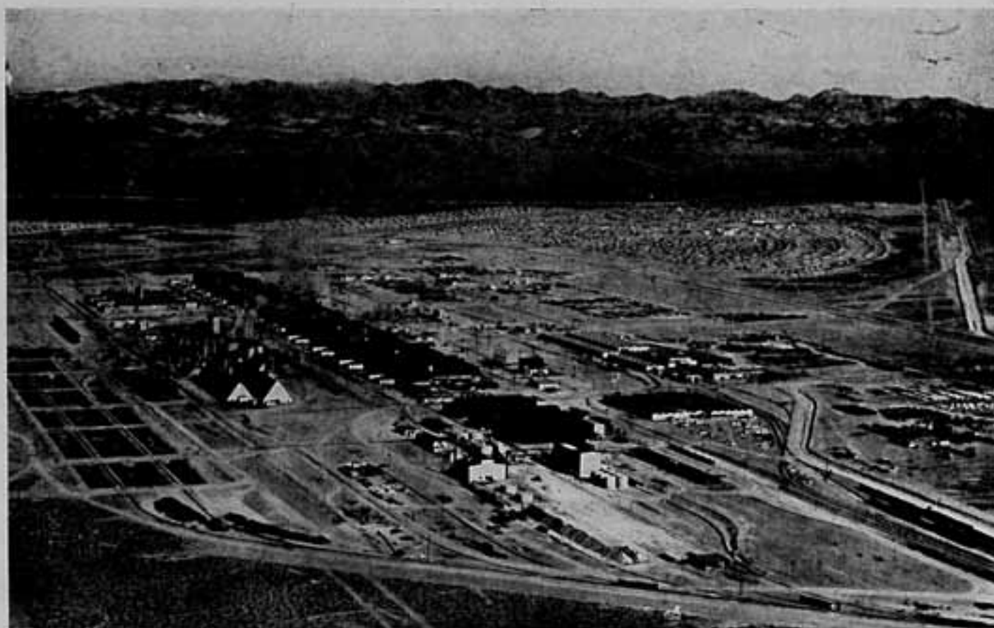
Fig. 3.—An aerial view of the large plant designed and built by Magnesium Elektron Limited for the United States Government. This plant, designed to produce 50,000 tons per annum, produced its first metal ten months from the day the ground was broken.
